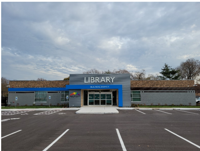
Mid-Continent Public Library’s renovated Blue Ridge Branch
